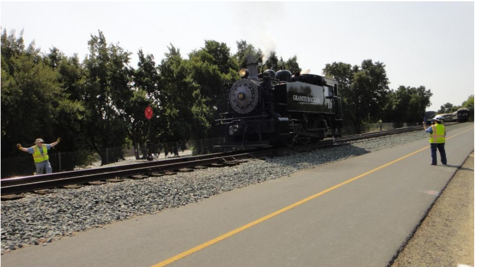
Granite Rock No. 10 passes through the MOW work-limits on its 11 o'clock run-around
