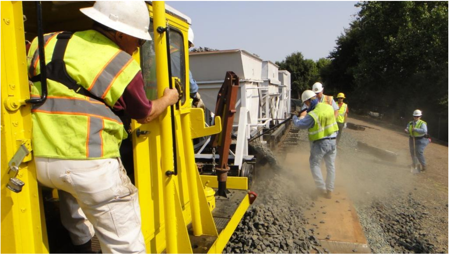
Mike H. pilots the tug as Mike M. and Chris C. drop rock onto the plywood which will then be shoveled over to build up the bank
