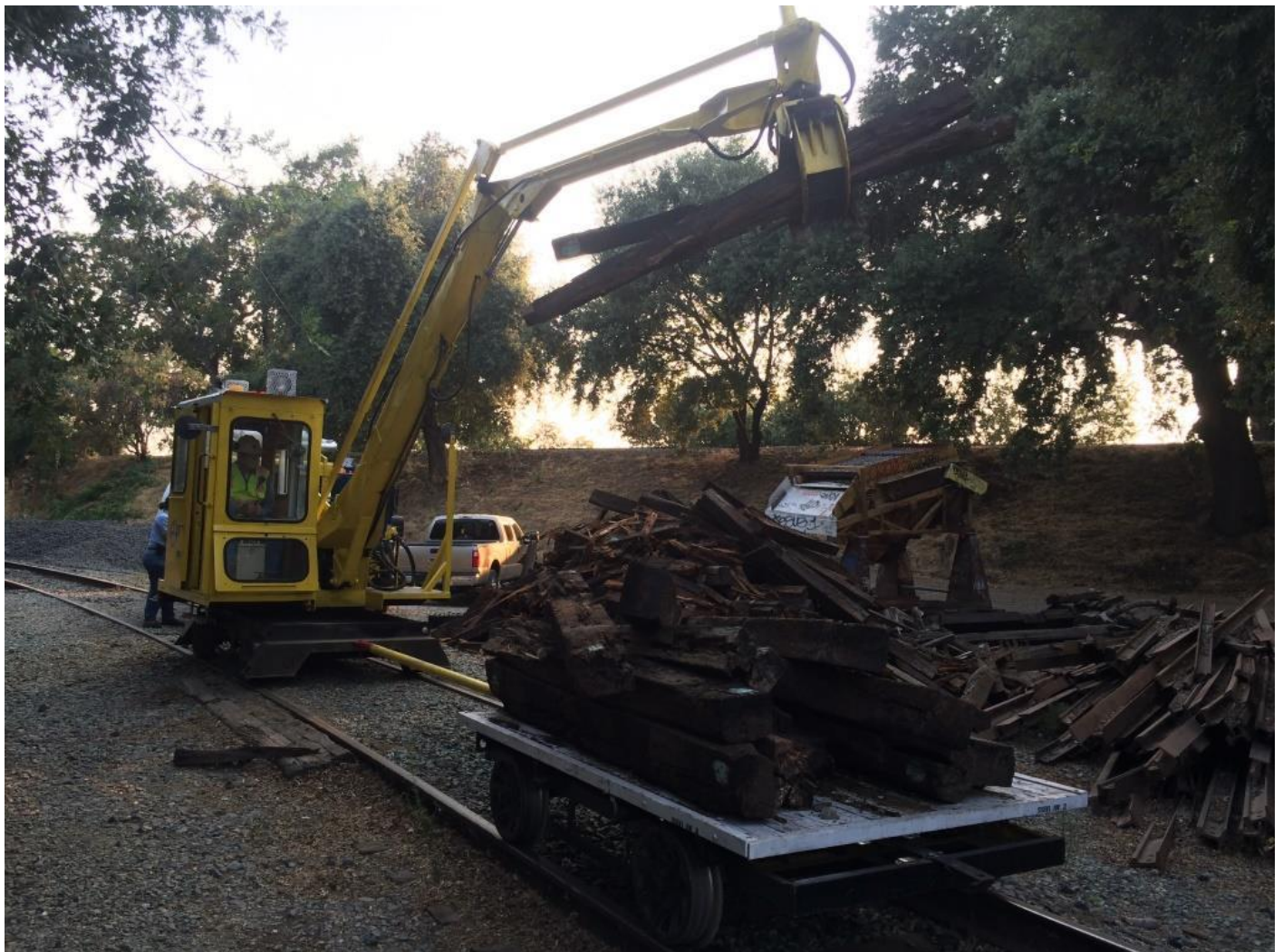
It's alive! Finally, after about four hours of work, the tie-crane fired right up
