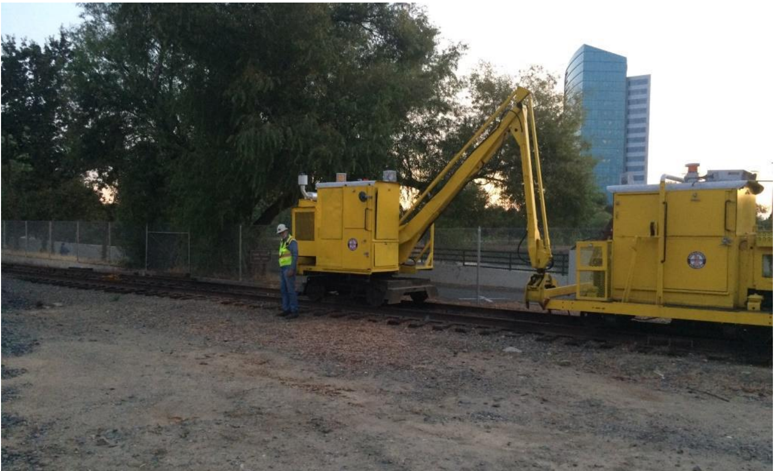
Finally, at 8:34 p.m., the tie-crane is put to bed...
