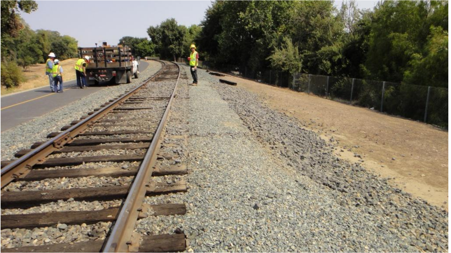
Chris M. surveys the completed Phase-1 of the project. The east-bank has been built up to help stop erosion
