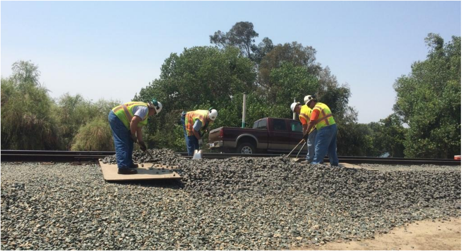
After lunch, Phase 2 of the project was tackled: the area around the switch stand
