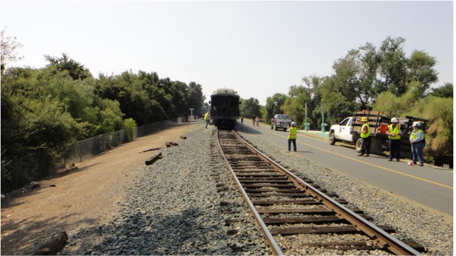
Brakeman Mike Reed steps off the train onto the newly reinforced brakeman landing-strip
