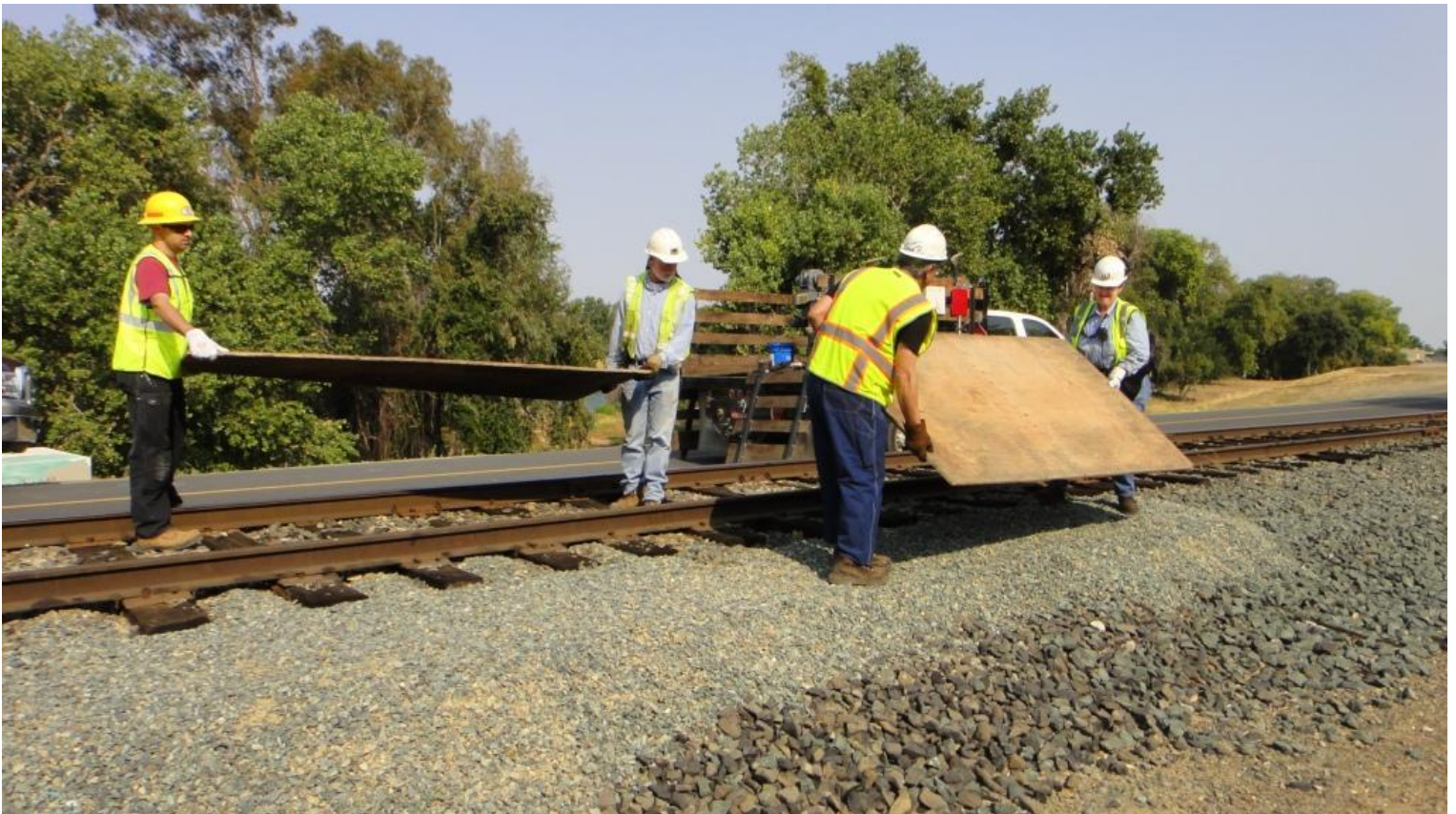
To the north of Switch 17 at Baths, Chris M., Mike M., John, and Heather place plywood sheets over the fine rock on the landing-strip
