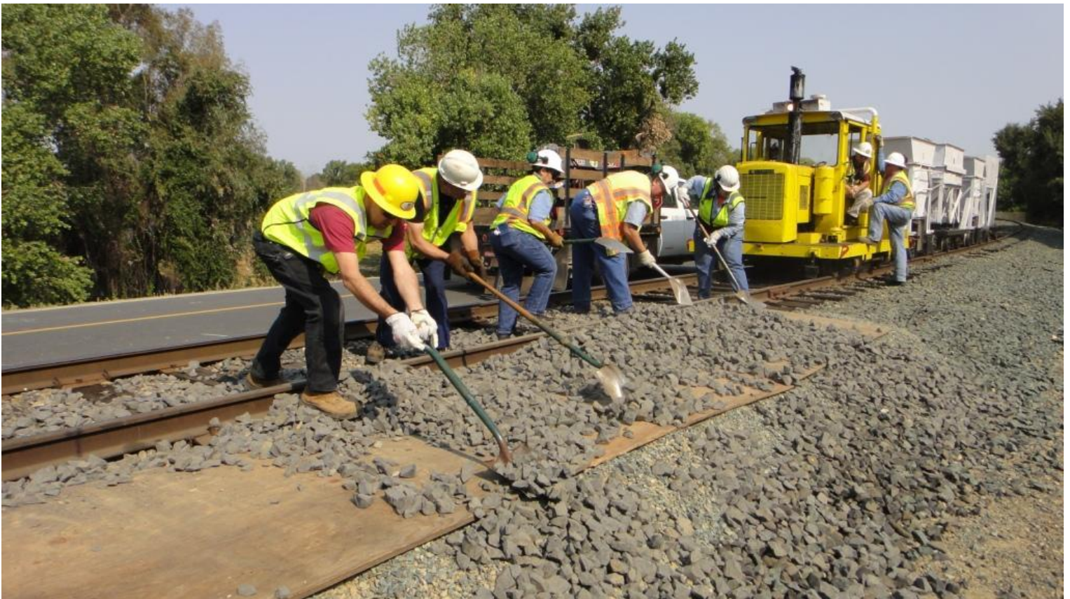
Chris M., John, Pam, Chris C., and Heather start moving rock across the plywood to build-up the bank of along the brakeman landing strip
