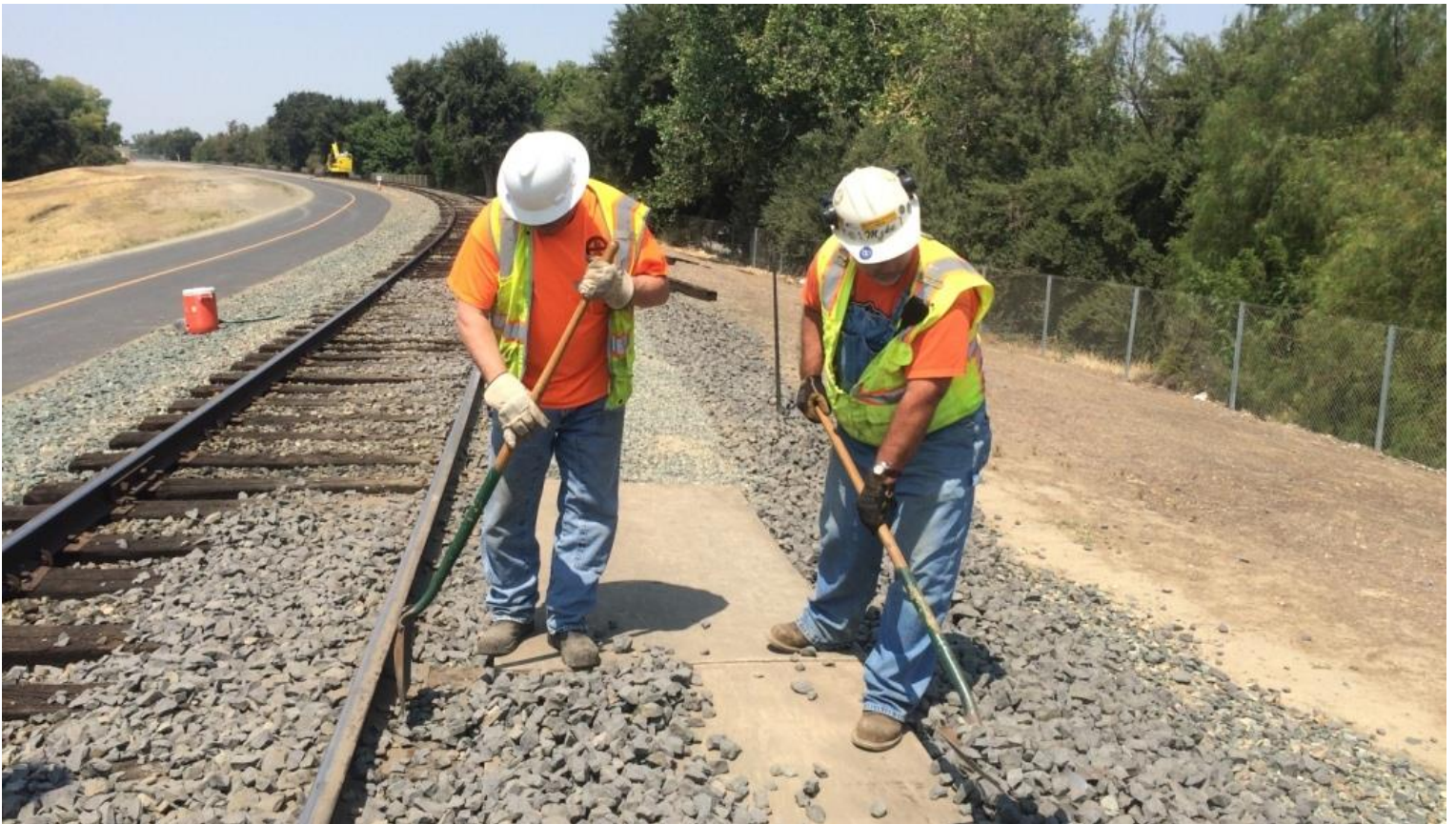
Scott and Mike F. build-up the bank around the switch stand
